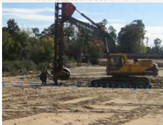
Wick Drains & Surcharge Accelerated Settlement
